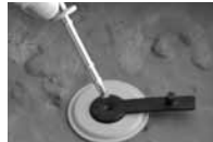
Remove rod after concrete hardens
